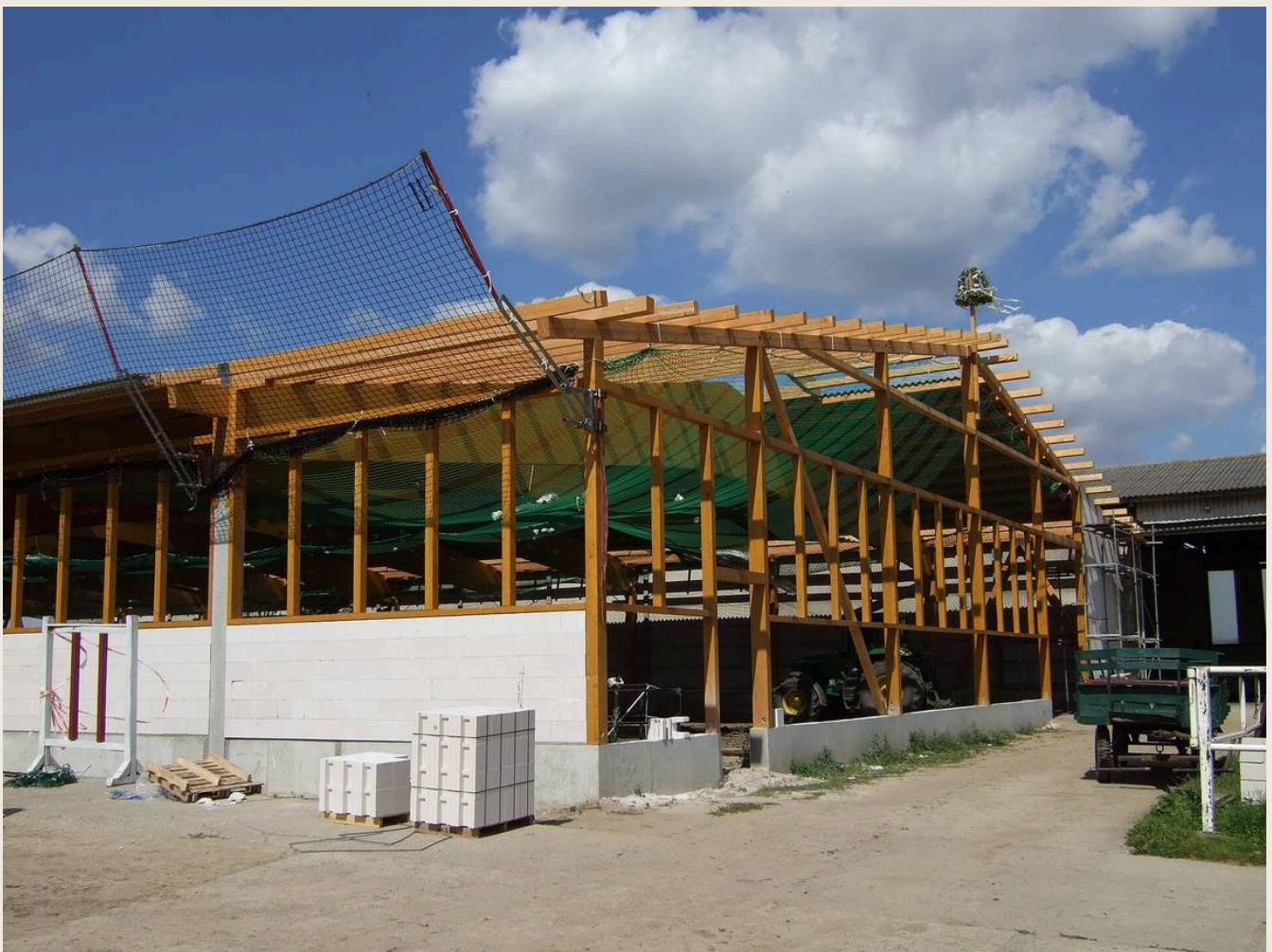
A site-built ADU starts as a frame: the stage where position, plumbing runs and window sizes are still cheap to change. Source: "Modern timber framing in pritzenhagen germany" by Sebastian Wallroth, via Wikimedia Commons — Public domain. Source and licence
