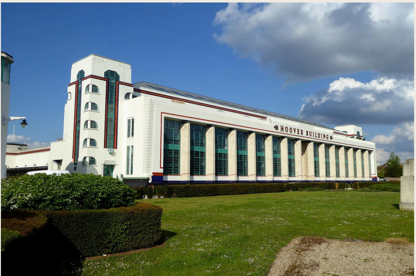
FIG. 09 · HOOVER BUILDING, PERIVALE, LONDON · PHOTO: ETHAN DOYLE WHITE / WIKIMEDIA COMMONS, CC BY-SA 4.0 · RESIZED. Source and licence
