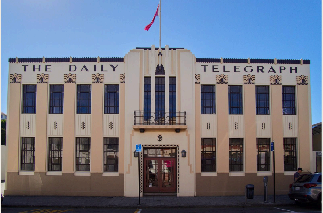
FIG. 08 · DAILY TELEGRAPH BUILDING, NAPIER · PHOTO: LUMOPLANK / WIKIMEDIA COMMONS, CC0 · RESIZED. Source and licence
