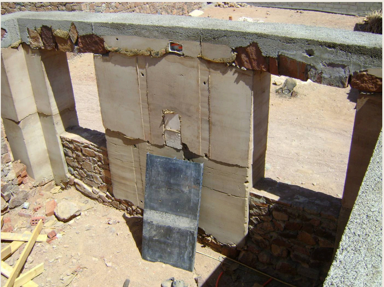
FIG. 11 · A RAMMED EARTH WALL UNDER CONSTRUCTION — A LOW-CARBON MATERIAL LEVER · PHOTO: Moshirah / WIKIMEDIA COMMONS · CC BY-SA 3.0. Source and licence
