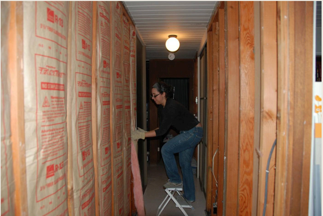
FIG. 09 · WALL INSULATION BEING INSTALLED — OPERATIONAL AND EMBODIED CARBON MEET IN THE ENVELOPE · PHOTO: Nick Nguyen / WIKIMEDIA COMMONS · CC BY-SA 2.0. Source and licence
