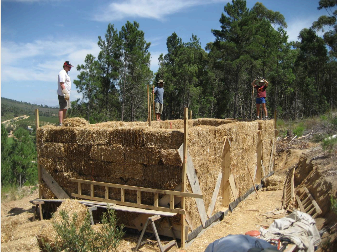
FIG. 12 · A STRAW-BALE HOUSE UNDER CONSTRUCTION · PHOTO: philipp / WIKIMEDIA COMMONS · CC BY 2.0. Source and licence
