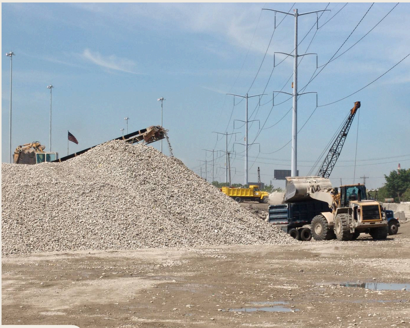
Skip to main content · D RECYCLED CONCRETE AGGREGATE — WHAT DEMOLITION CAN BECOME · PHOTO: ChicagoConcrete / WIKIMEDIA COMMONS · CC BY-SA 3.0. Source and
