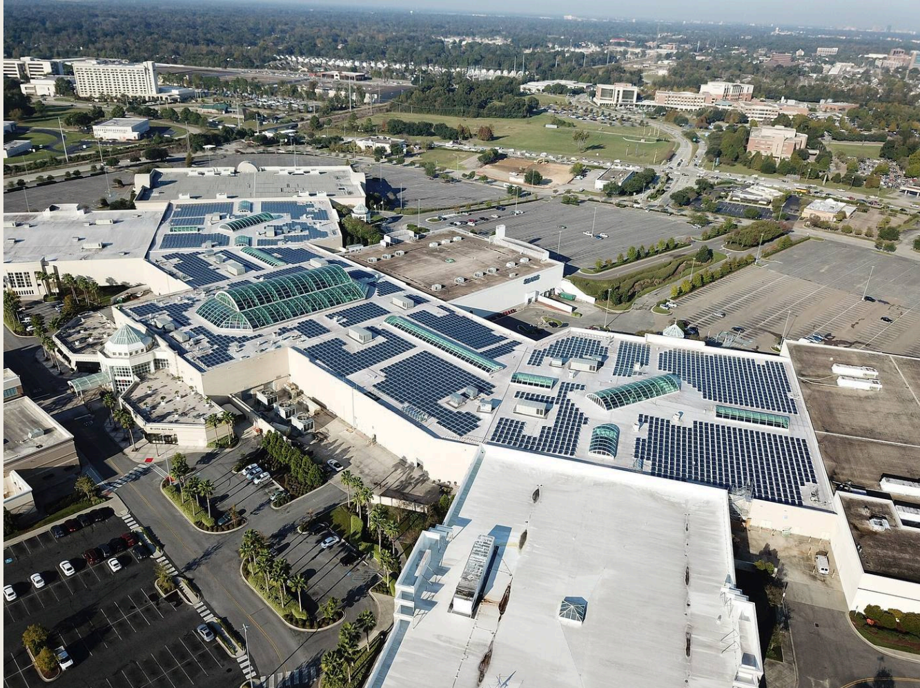
FIG. 08 · SOLAR PV ON A LARGE FLAT ROOF · PHOTO: JDCANTIN / WIKIMEDIA COMMONS · CC BY-SA 4.0. Source and licence
