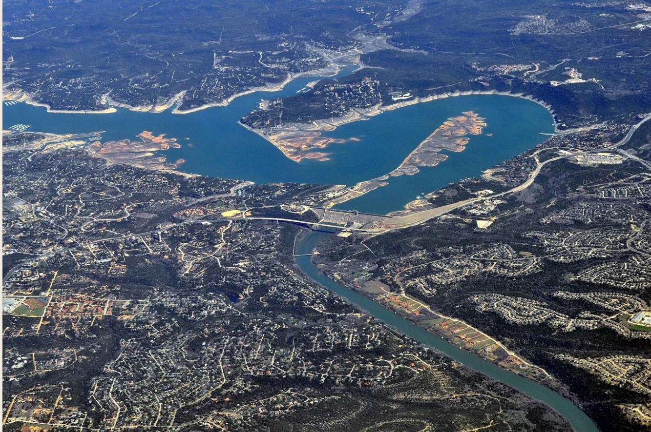
FIG. 11 · MANSFIELD DAM AND LAKE TRAVIS · PHOTO: JOE MABEL / WIKIMEDIA COMMONS · CC BY 3.0. Source and licence
