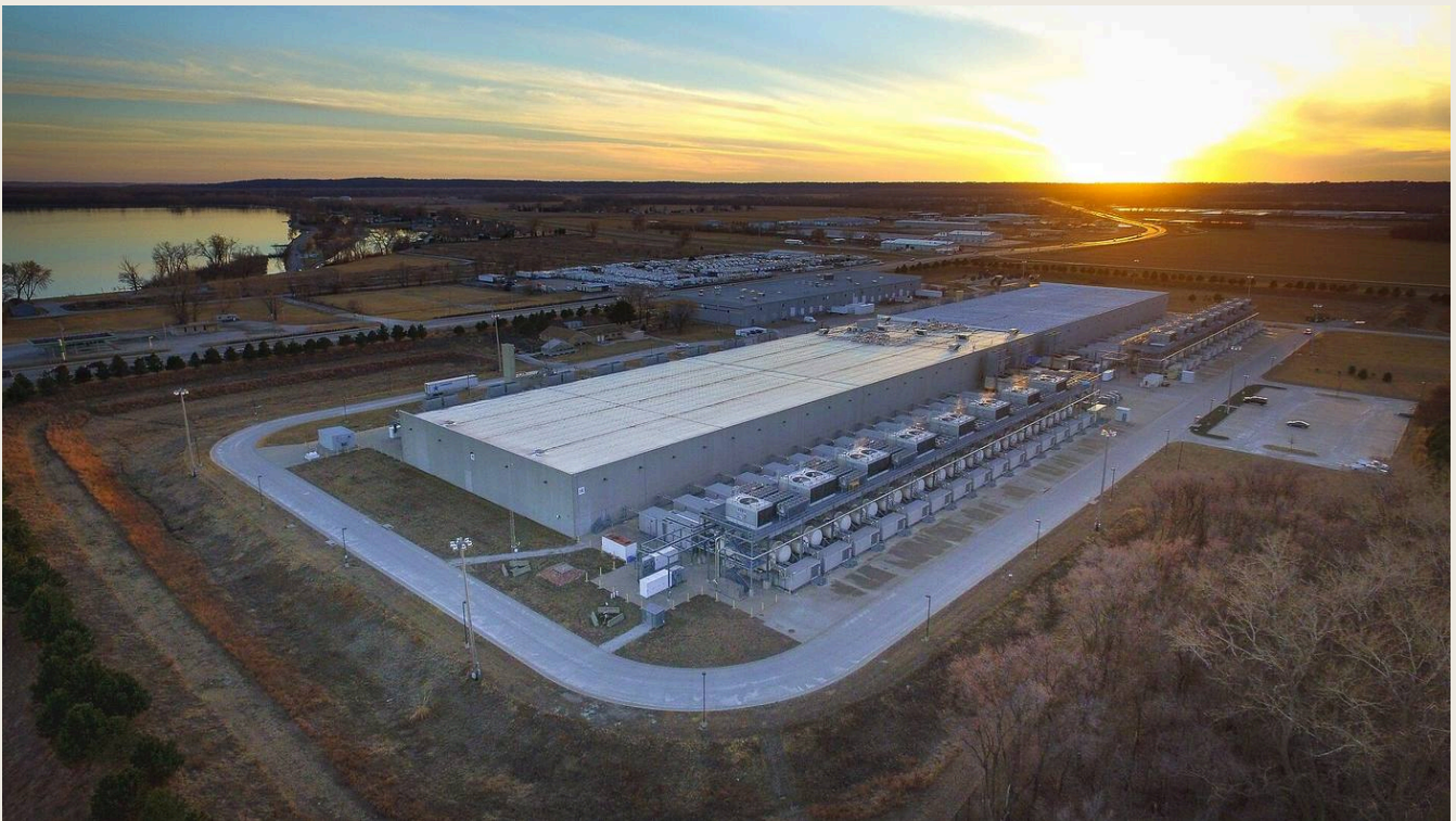
FIG. 15 · DATA-CENTRE CAMPUS, COUNCIL BLUFFS, AT SUNSET · PHOTO: CHAD DAVIS / WIKIMEDIA COMMONS · CC BY 2.0. Source and licence
