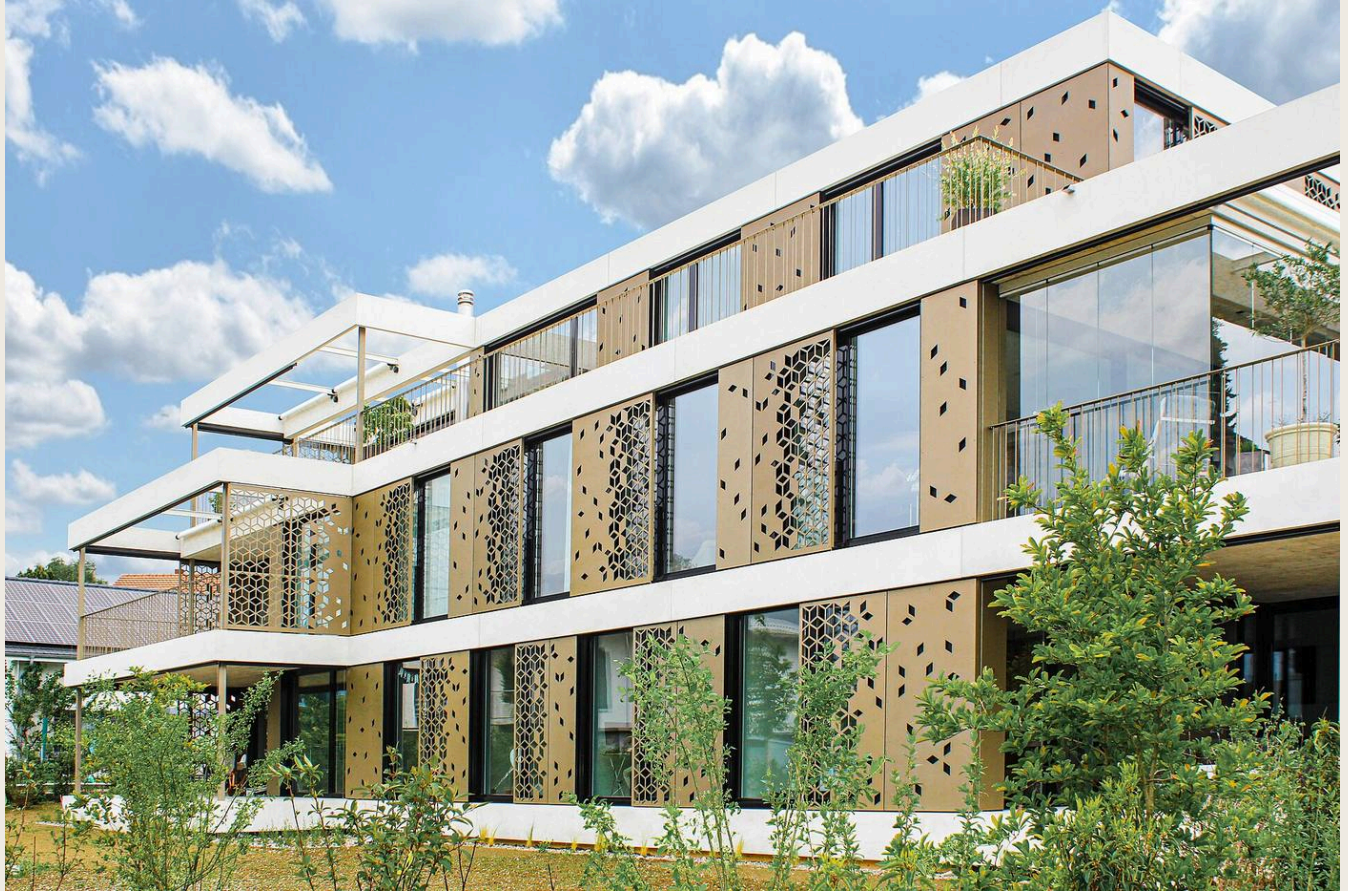
FIG. 06 · PERFORATED METAL SHADING SCREEN, BELLMUND · PHOTO: NINA ZÜLLIG / WIKIMEDIA COMMONS · CC BY 4.0. Source and licence
