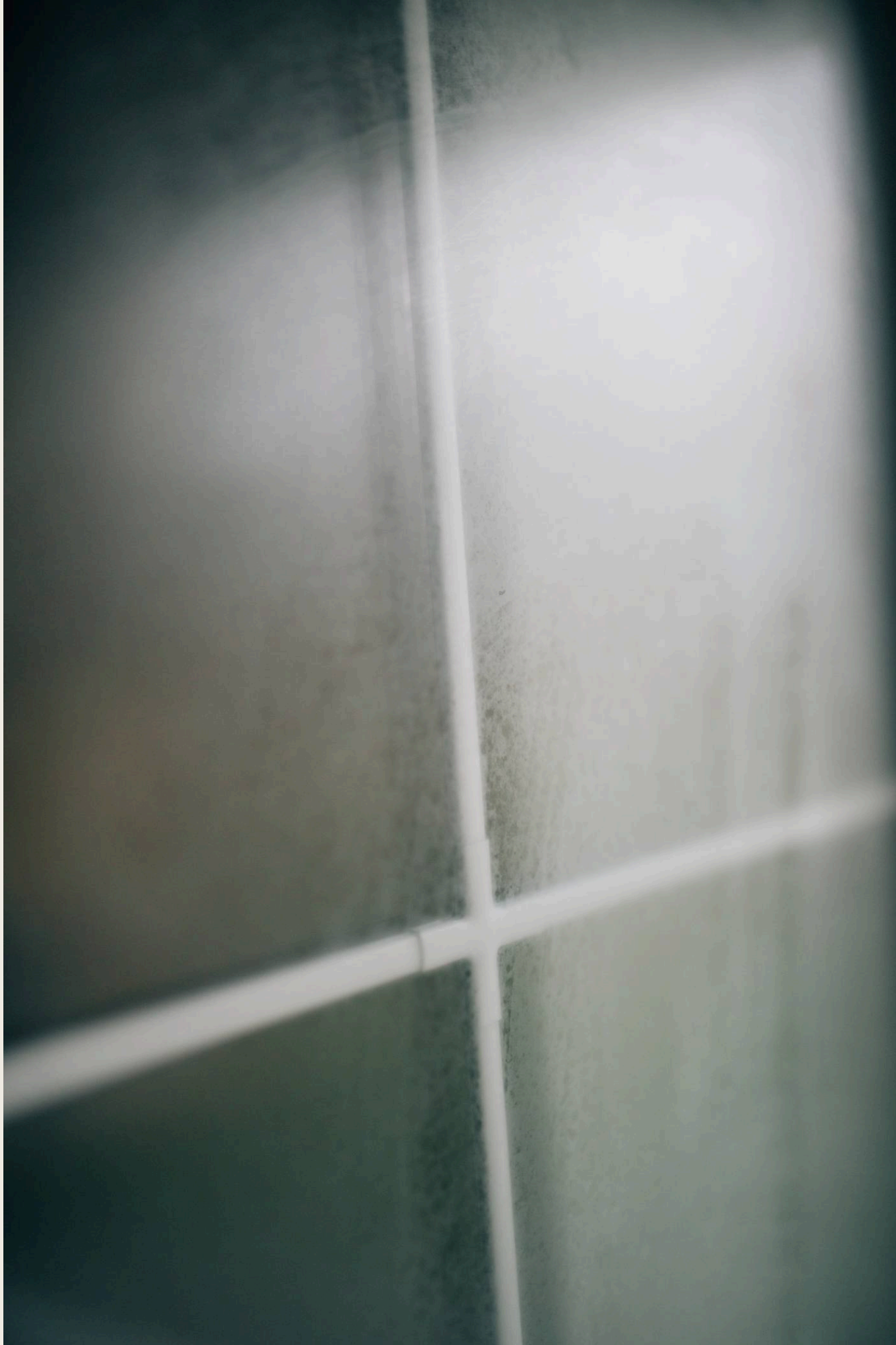
FIG. 02 · CONDENSATION DROPLETS ON GLASS · PHOTO: Shixart1985 / WIKIMEDIA COMMONS · CC BY 2.0. Source and licence
