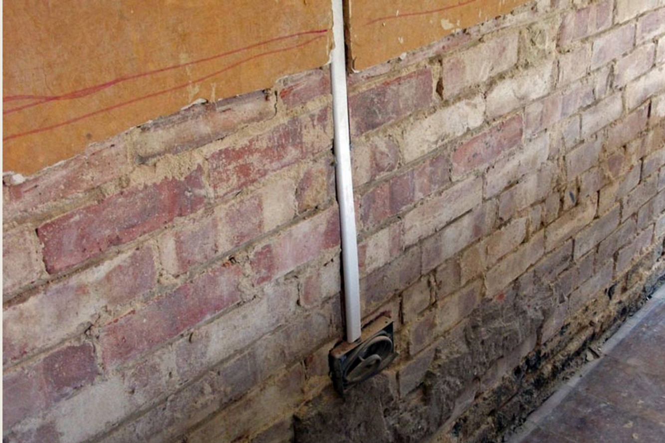
FIG. 09 · PLASTER REMOVED FOR RISING-DAMP INSPECTION · PHOTO: Kebabknight / WIKIMEDIA COMMONS · CC BY-SA 3.0. Source and licence
