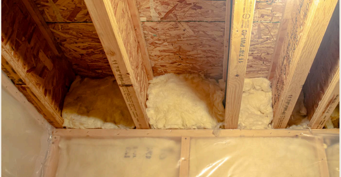
FIG. 02 · ENGINEERED I-JOIST IN A BASEMENT · PHOTO: WIKIDEAS1 / WIKIMEDIA COMMONS · CC0 1.0. Source and licence
