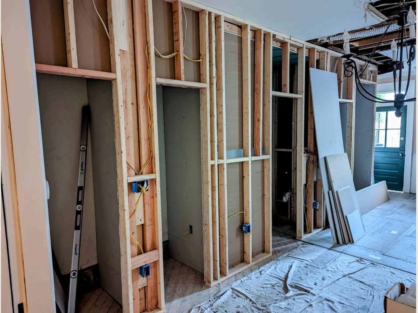
FIG. 01 · TIMBER STUD WALL FRAMING EXPOSED DURING A HOME RENOVATION · PHOTO: KURTKAISER / WIKIMEDIA COMMONS · CC0 1.0. Source and licence
