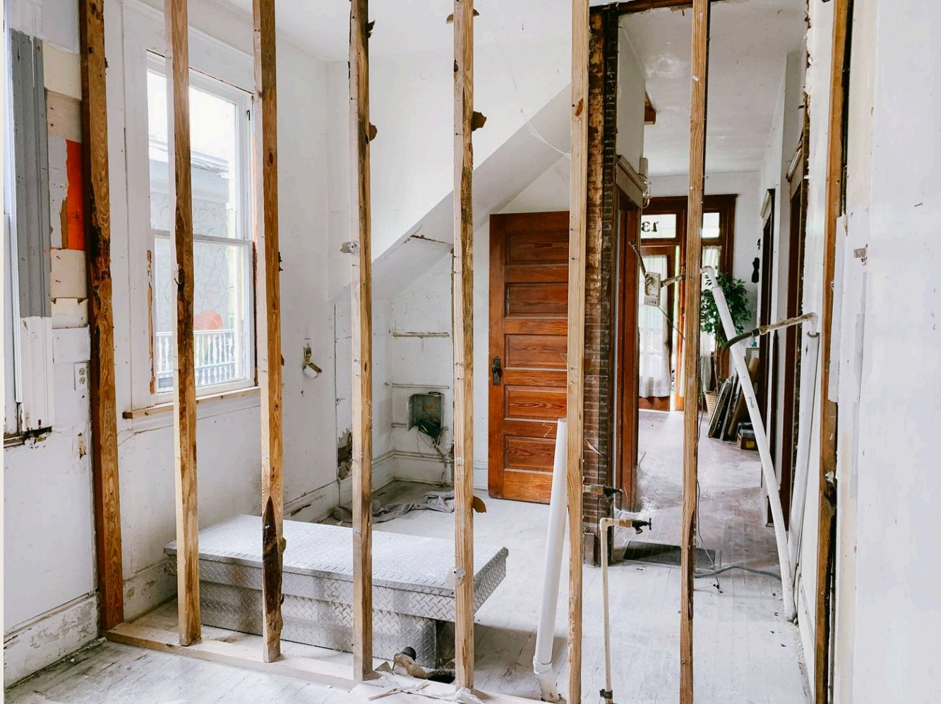
FIG. 03 · EXPOSED TIMBER WALL STUDS IN A HOME UNDER RENOVATION · PHOTO: MONICA SILVESTRE / PEXELS · FREE LICENCE. Source and licence
