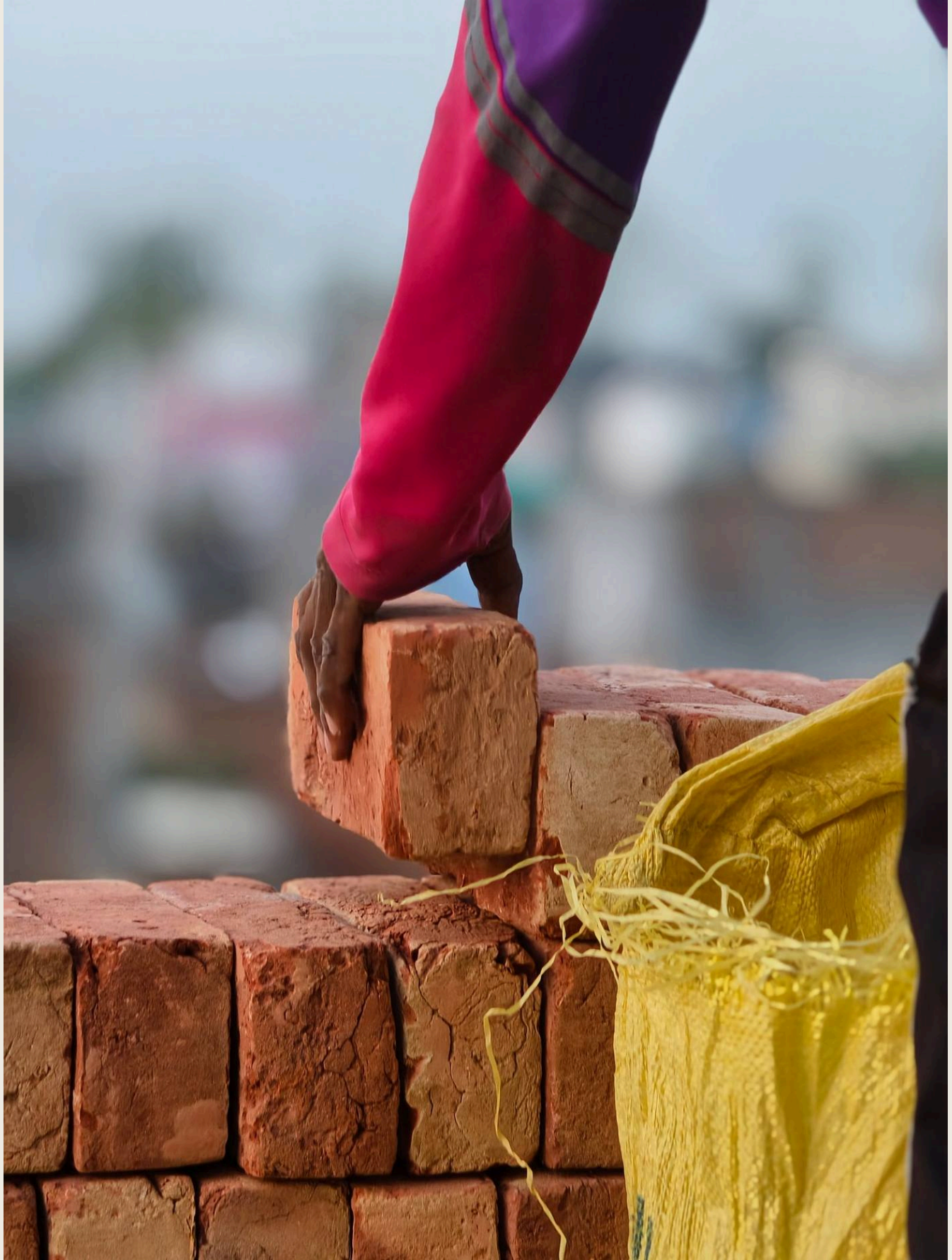
FIG. 05 · A WORKER PLACING A BRICK DURING WALL CONSTRUCTION · PHOTO: VIKESH ZEN / PEXELS · FREE LICENCE. Source and licence
