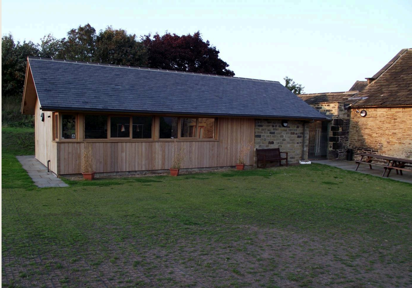
FIG. 01 · NORTHORPE HALL, YORKSHIRE — A TIMBER-CLAD REAR EXTENSION ON A STONE BUILDING · PHOTO: Chris Pattinson / WIKIMEDIA COMMONS · CC BY-SA 2.0. Source and licence
