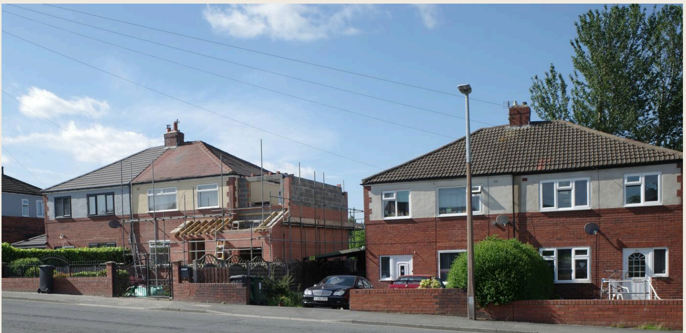
FIG. 09 · EXTENSION UNDER CONSTRUCTION, LIVERSEEDGE · PHOTO: habiloid / WIKIMEDIA COMMONS · CC BY-SA 2.0. Source and licence
