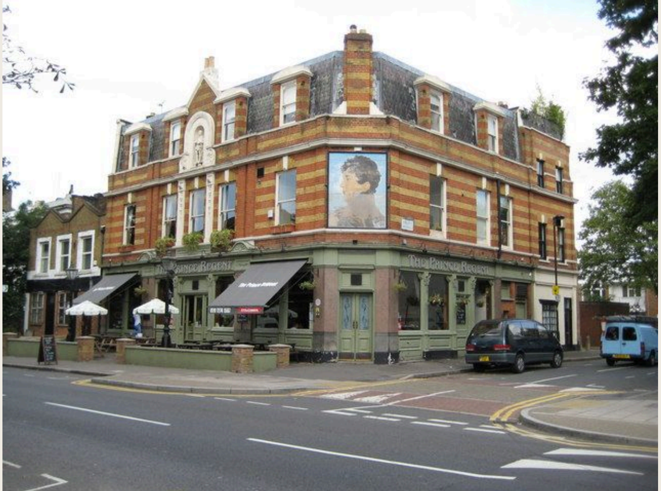
FIG. 01 · THE PRINCE REGENT, HERNE HILL — MANSARD ROOF AND DORMERS · PHOTO: NIGEL COX / WIKIMEDIA COMMONS · CC BY-SA 2.0. Source and licence
