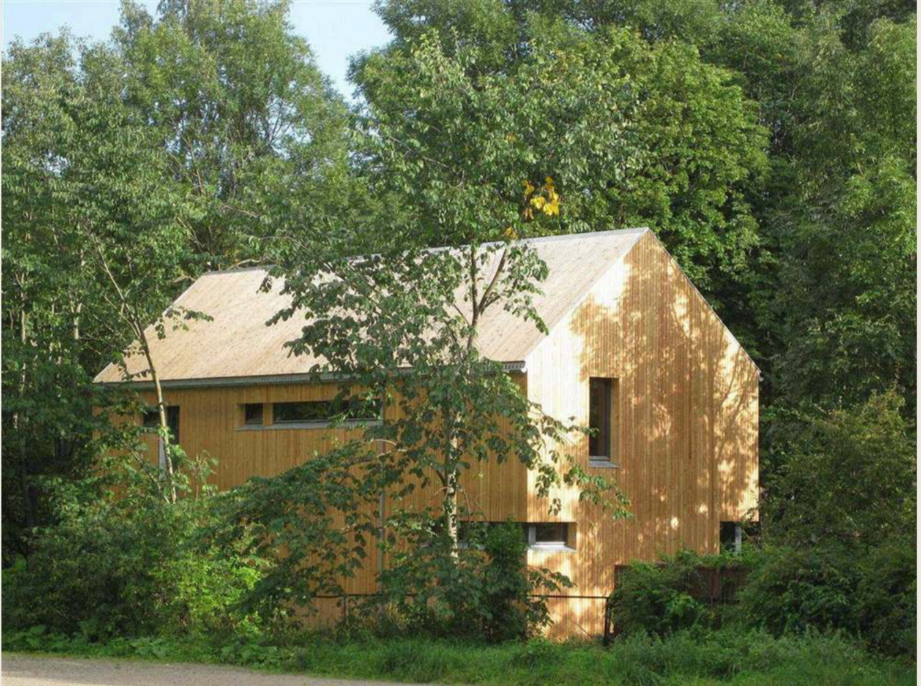
FIG. 01 · PASSIVE HOUSE, LADEVEIEN, OSLO · PHOTO: STEIN STOKNES / WIKIMEDIA COMMONS, CC BY 3.0 · RESIZED.
