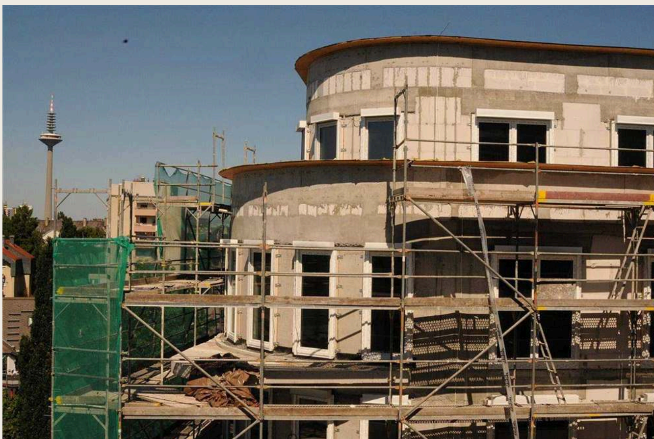
FIG. 04 · PASSIVE HOUSE CONSTRUCTION, FRANKFURT · PHOTO: SUSANA SECRETARIAT / WIKIMEDIA COMMONS, CC BY 2.0 · RESIZED.
