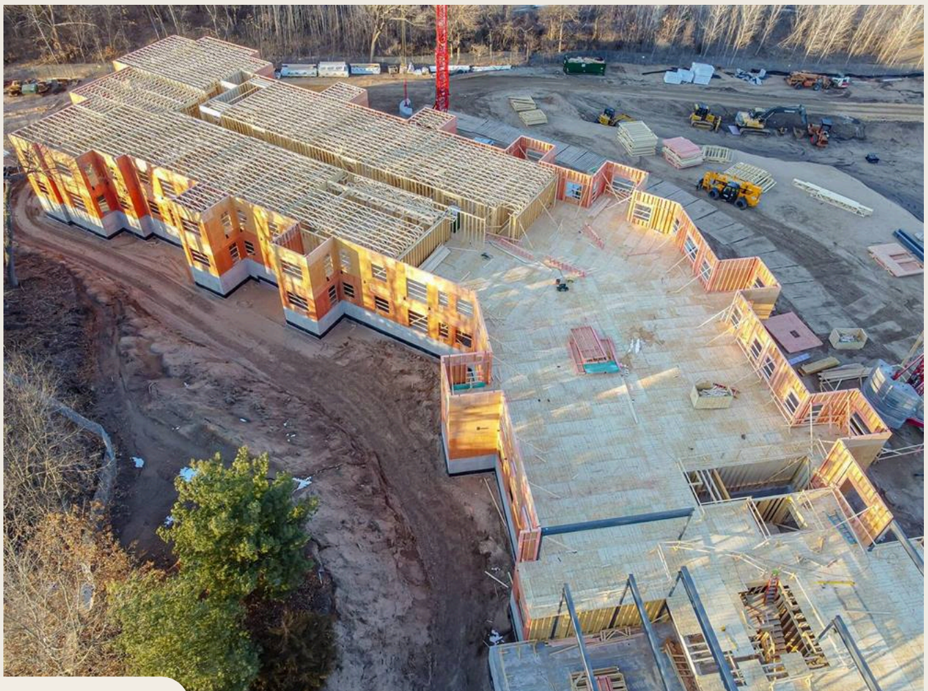
Skip to main content · PREFABRICATED FRAMING ON SITE · PHOTO: WIKIDEAS1 / WIKIMEDIA COMMONS, CC0 1.0 · LOCALLY HOSTED RESIZE. Photo source and licence
