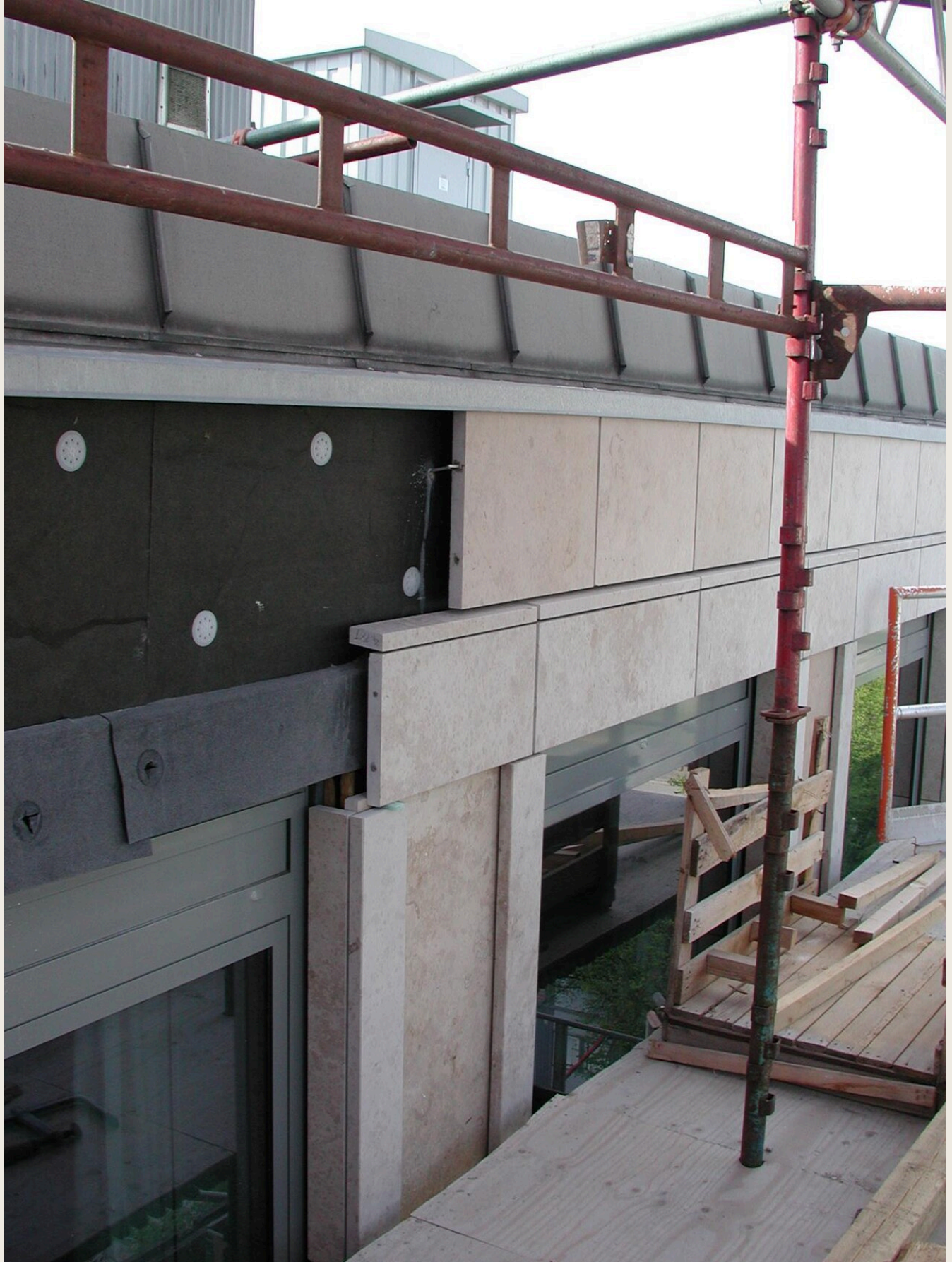
FIG. 03 · VENTILATED LIMESTONE FACADE INSTALLATION · PHOTO: J. STIEGLER / WIKIMEDIA COMMONS, CC BY-SA 3.0 · RESIZED.
