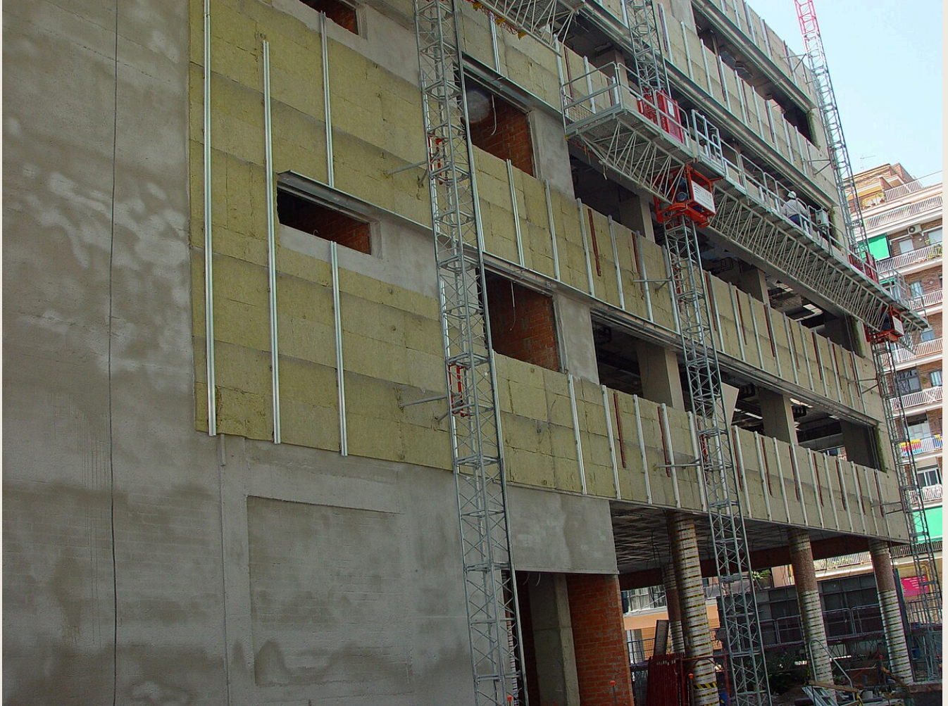
FIG. 04 · STONE-WOOL INSULATION BEHIND A VENTILATED FACADE · PHOTO: ENGOMAN23 / WIKIMEDIA COMMONS, PUBLIC DOMAIN · RESIZED.
