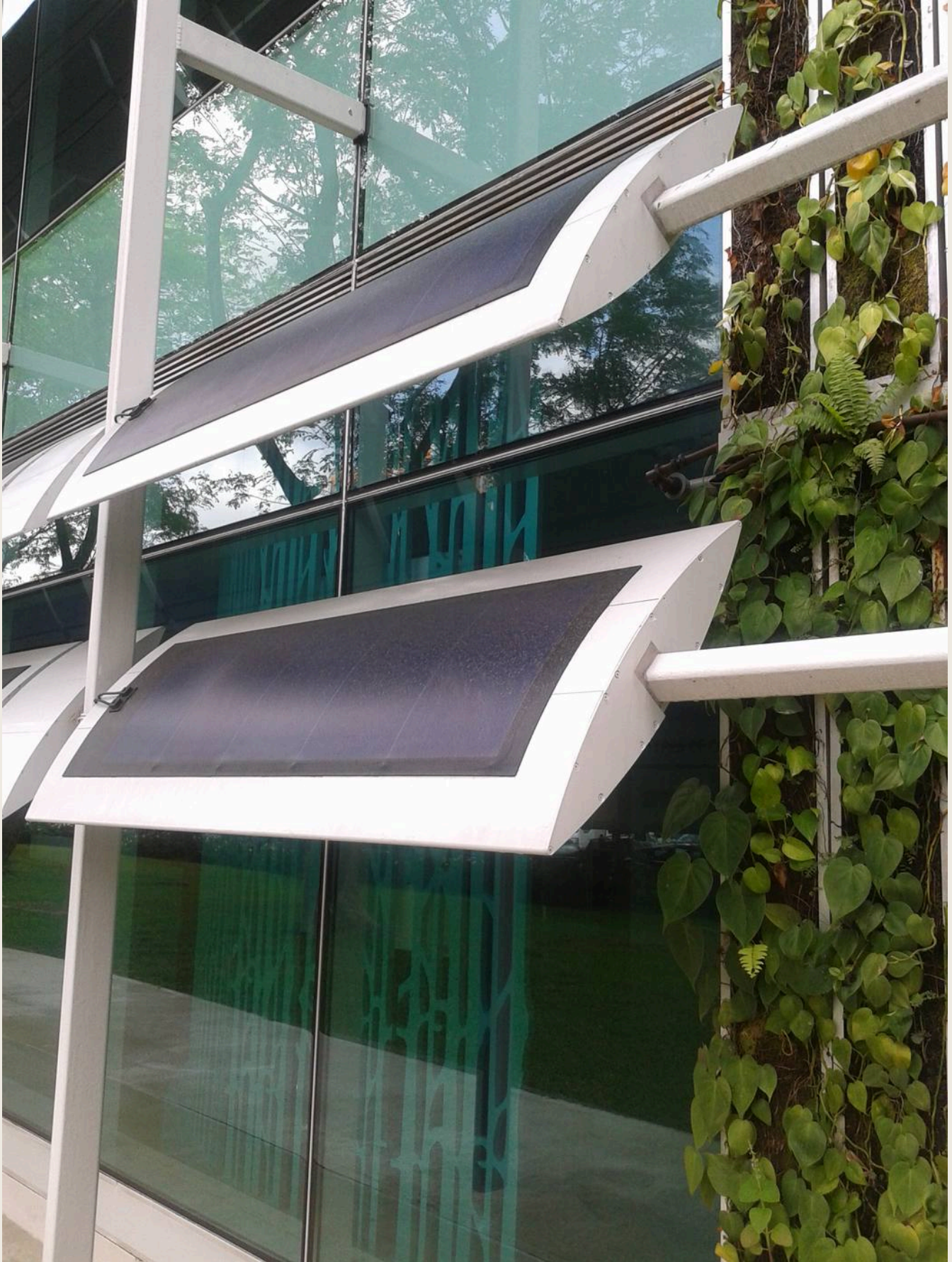
FIG. 07 · PV AS EXTERNAL SHADING FINS · PHOTO: Esmail7 / WIKIMEDIA COMMONS · CC BY-SA 3.0. Source and licence
