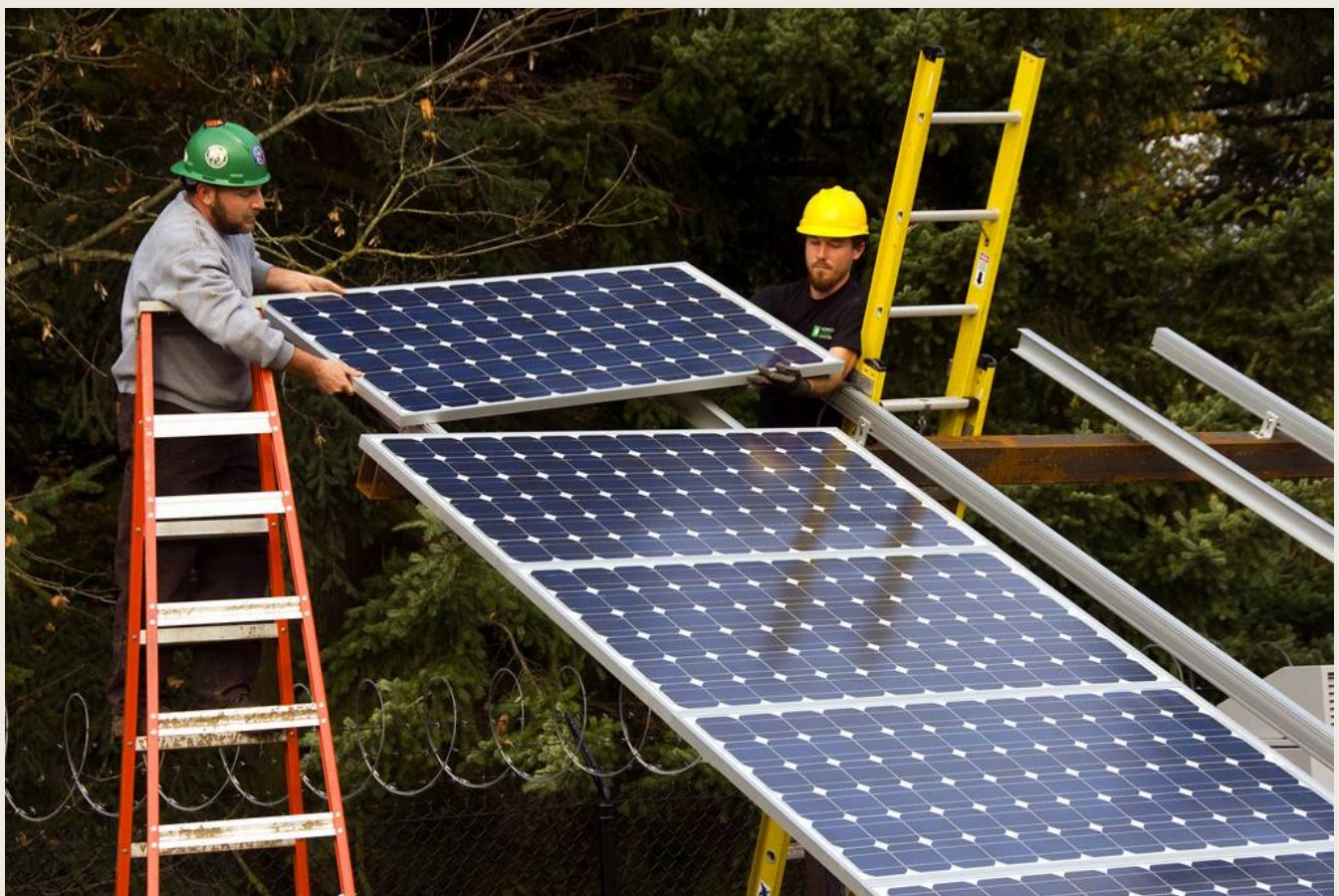
FIG. 10 · INSTALLING PV MODULES · PHOTO: Oregon Department of Transportation / WIKIMEDIA COMMONS · CC BY 2.0. Source and licence
