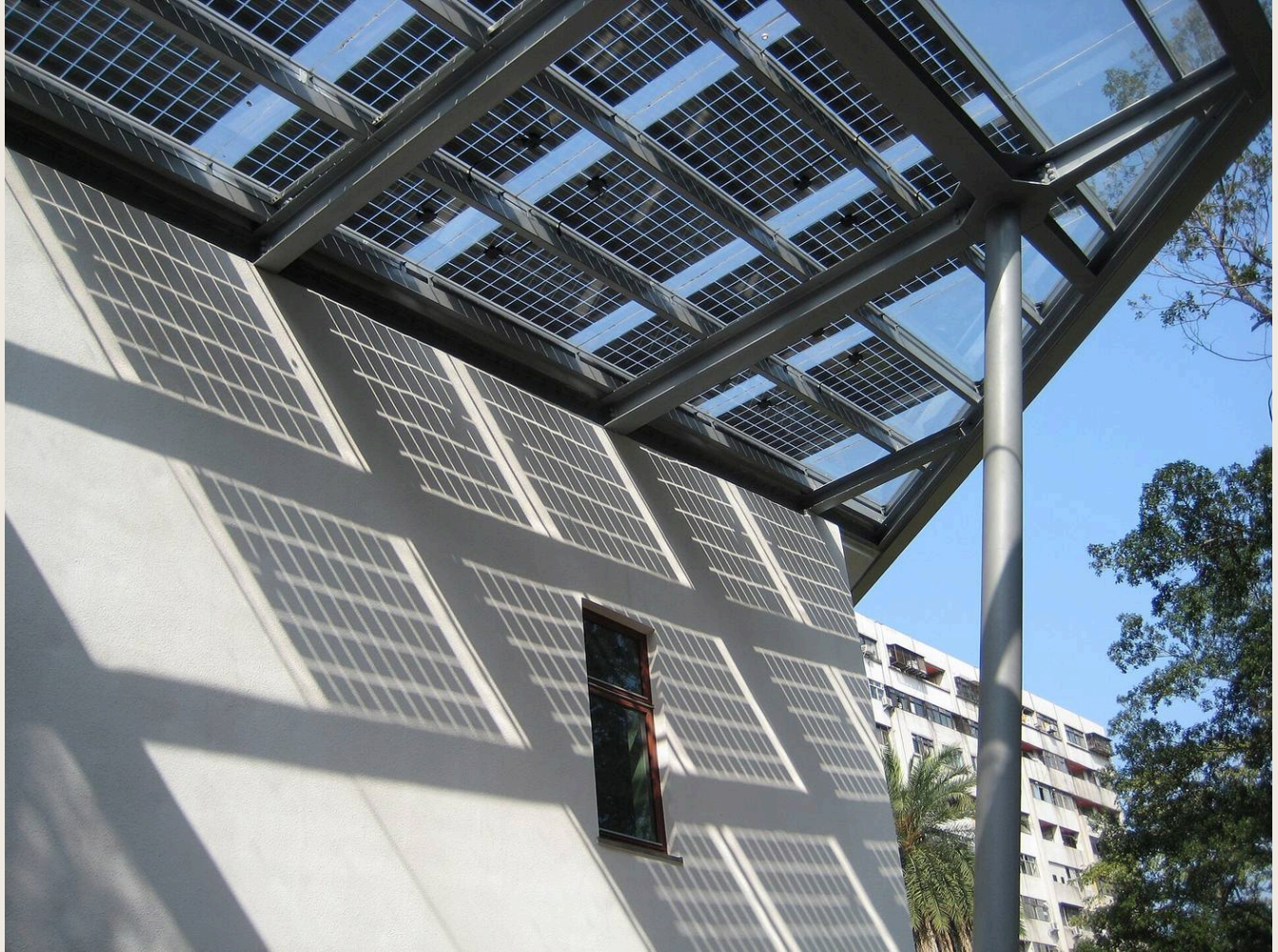
FIG. 04 · BIPV AS THE BUILDING SKIN IN TAIPEI · PHOTO: Littleha / WIKIMEDIA COMMONS · CC BY 2.5. Source and licence
