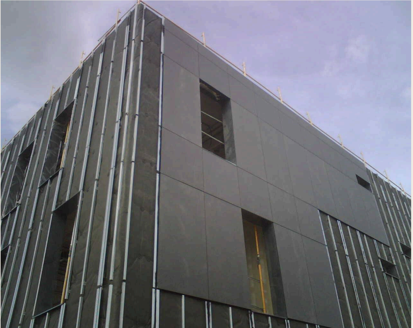
FIG. 06 · A VENTILATED RAINSCREEN BUILD-UP · PHOTO: Frankpulido / WIKIMEDIA COMMONS · PUBLIC DOMAIN. Source and licence
