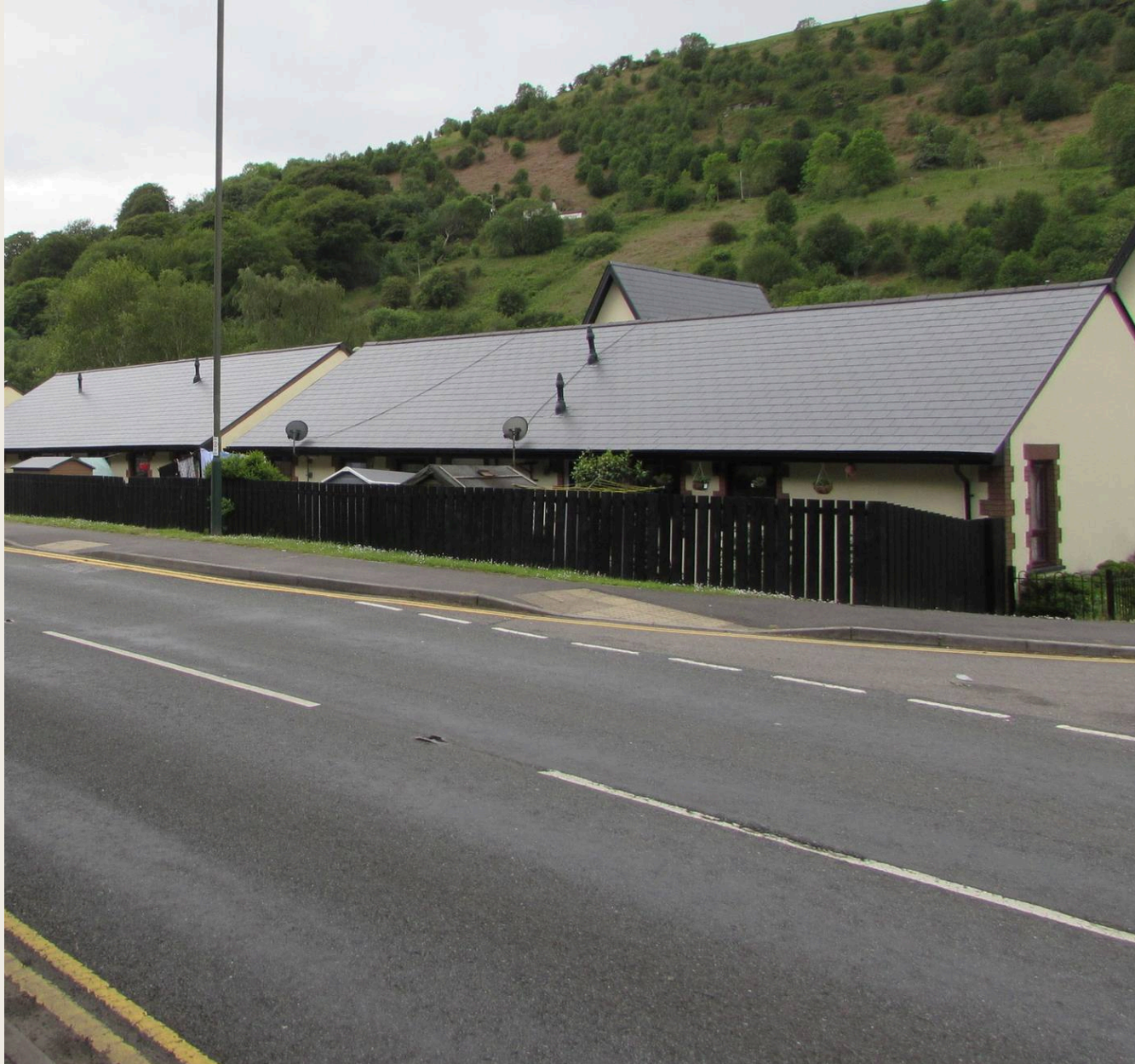
FIG. 11 · LOW-PITCHED ROOFS AT RHOSYN GWYN, WALES — COMPACT FORMS, DURABLE MATERIALS · PHOTO: Jagger / WIKIMEDIA COMMONS · CC BY-SA 2.0. Source and licence
