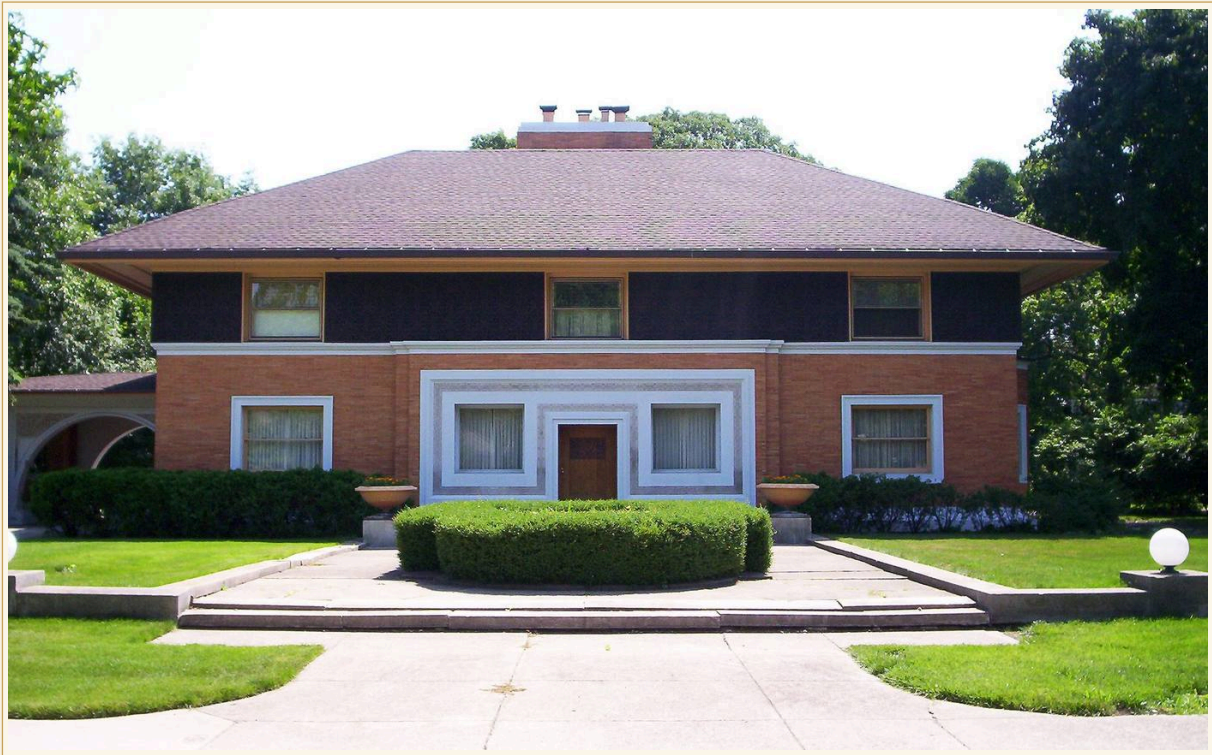
Photo: Oak Park Cycle Club, via Wikimedia Commons (CC BY-SA 2.0). Source: https://commons.wikimedia.org/wiki/File:William_H._Winslow_House_Front_Facade.jpg
