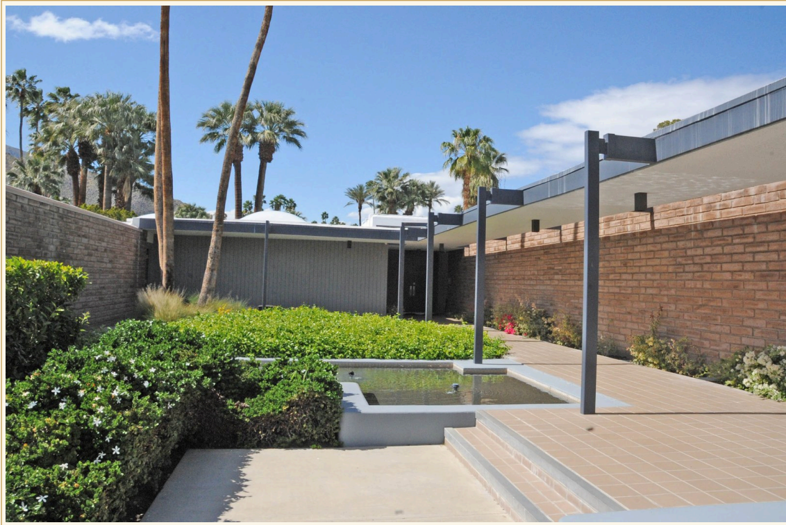
Photo: JERRY & ROY KLOTZ, M.D., via Wikimedia Commons (CC BY-SA 4.0). Source: https://commons.wikimedia.org/wiki/File:MAURICE_SMITH_AND_DINAH_SHORE_HOUSE_RIVERSIDE_COUNTY_CA.jpg
