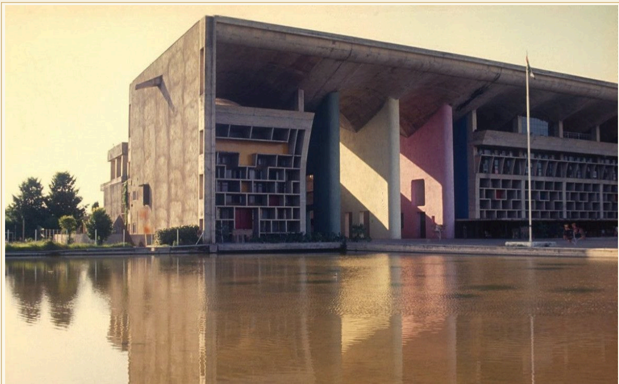
Photo: Nicholas.iyadurai, via Wikimedia Commons (CC BY-SA 4.0). Source: https://commons.wikimedia.org/wiki/File:Chandigarh_Capitol_Complex_-_Le_Corbusier_-_Highcourt_-_front_elevation.jpg
