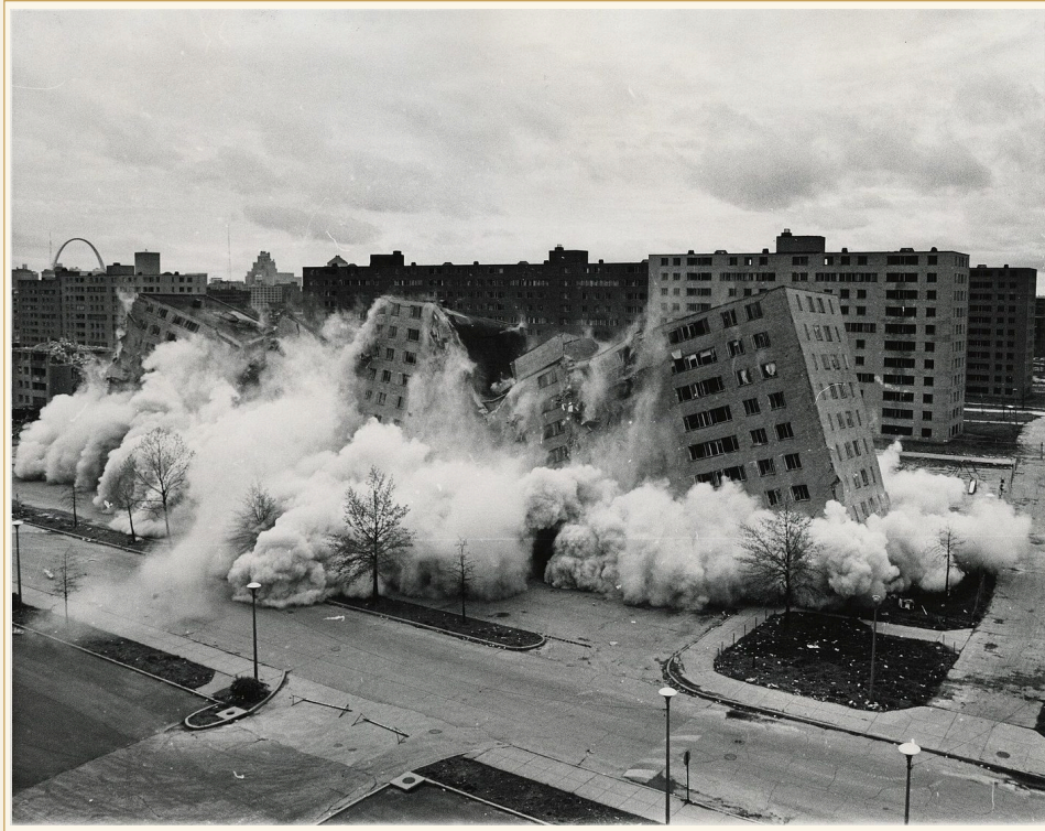
Photo: U.S. Department of Housing and Urban Development, via Wikimedia Commons (public domain). Source: https://commons.wikimedia.org/wiki/File:Pruitt-Igoe-collapses.jpg
