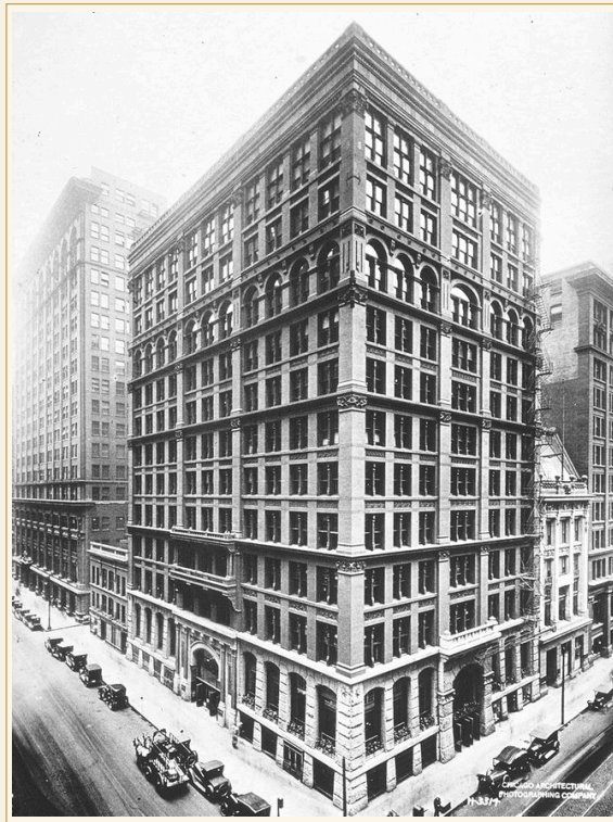
Photo: Chicago Architectural Photographing Company, via Wikimedia Commons (public domain). Source: https://commons.wikimedia.org/wiki/File:Home_Insurance_Building.JPG
