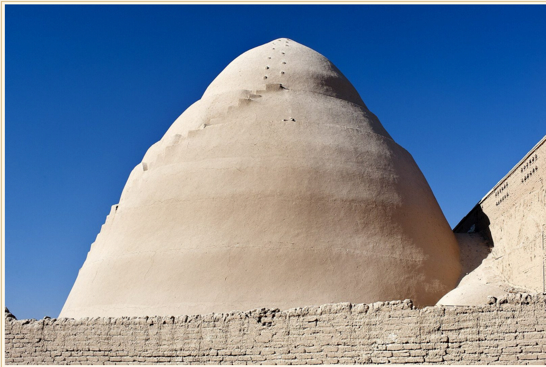
Photo: User:Ggia, via Wikimedia Commons (CC BY-SA 3.0). Source: https://commons.wikimedia.org/wiki/File:20110102_Ice_House_(exterior)_Meybod_Iran.jpg
