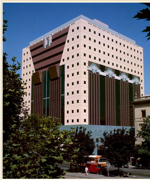
Photo: Steve Morgan, via Wikimedia Commons (CC BY-SA 3.0). Source: https://commons.wikimedia.org/wiki/File%3APortland%20Building%201982.jpg
