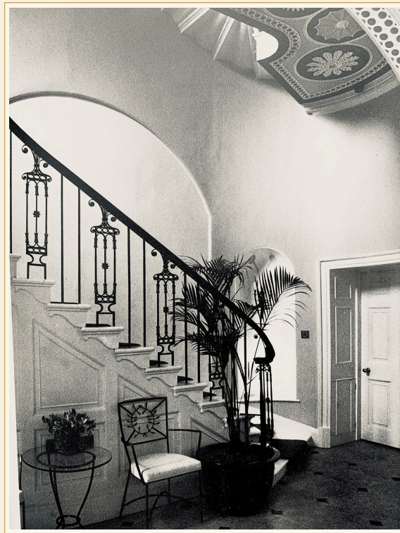
Photo: Georgian Boy 1776, via Wikimedia Commons (CC BY-SA 4.0). Source: https://commons.wikimedia.org/wiki/File:1_Bedford_Square,_London,_entrance_hall_and_staircase.jpg
