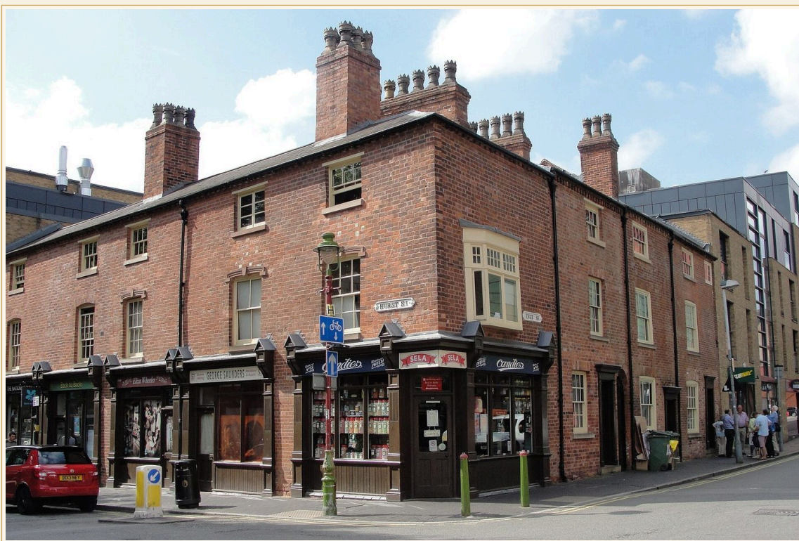
Photo: Nussy-Pic, via Wikimedia Commons (CC BY-SA 4.0). Source: https://commons.wikimedia.org/wiki/File:Back_to_Back,_Birmingham.JPG
