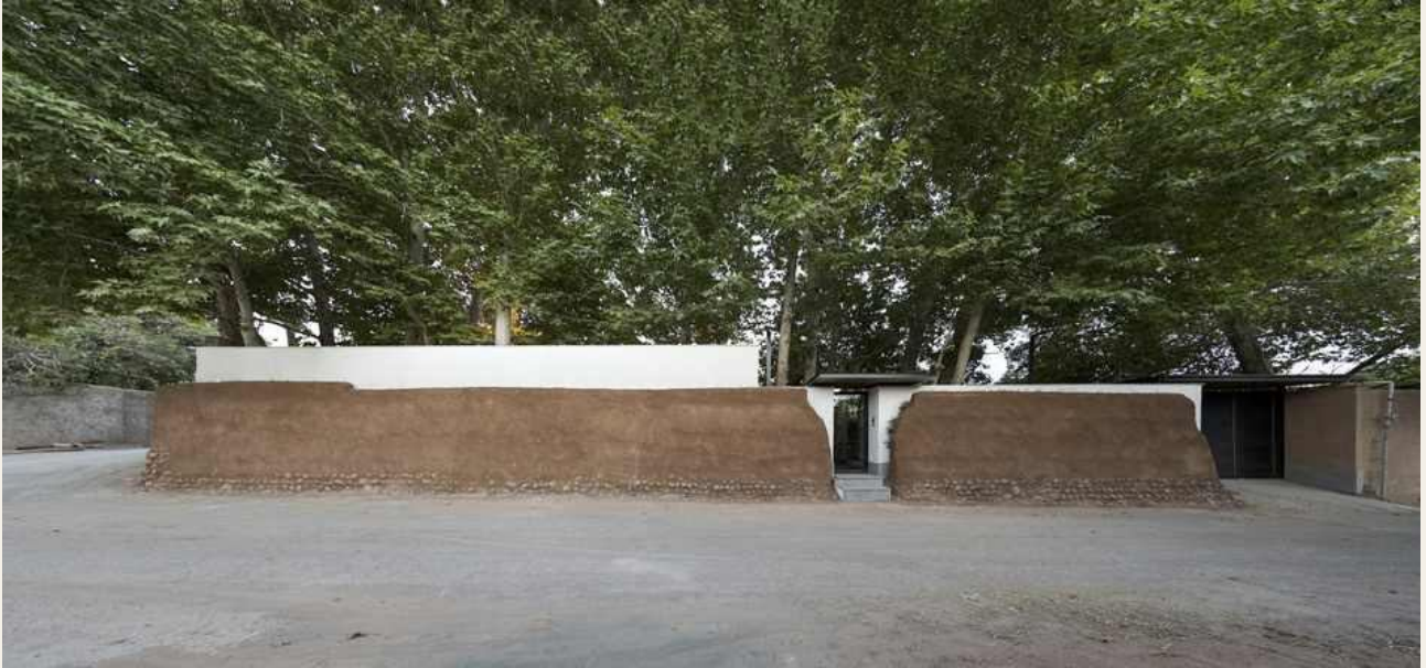
The retained garden boundary and renewed entrance
