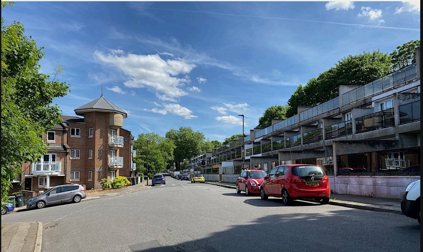
The Central Hill Estate, Crystal Palace (1967–75, Rosemary Stjernstedt) — saved from demolition with Cressingham Gardens. Photo: Robin Stott, via Geograph / Wikimedia Commons — CC BY-SA 2.0. Photo source ↗ · CC BY-SA 2.0
